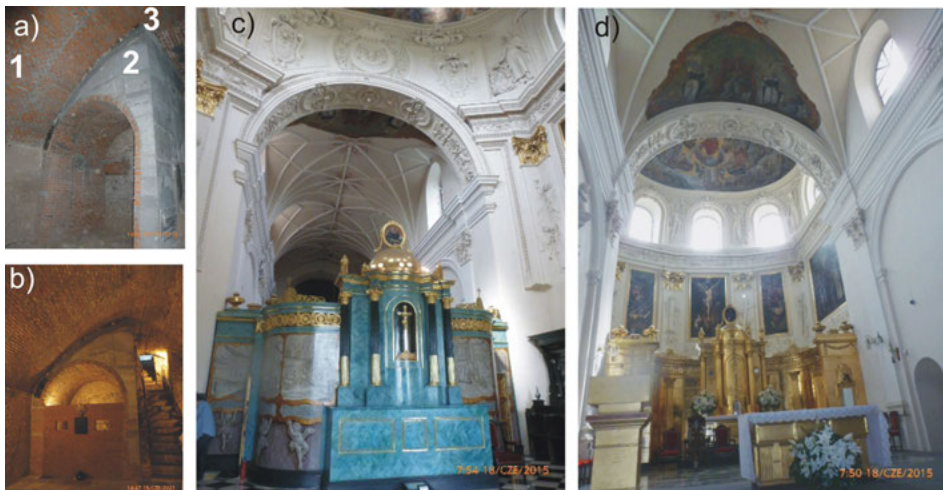
Fig. 10. The Tyszkiewicz chapel: a) and b) concrete structure in the crypt supporting the wide vault under the high altar, under construction and now (1 – rebuilt part of the vault, 2 – supporting concrete arch, 3 – original part of the vault), c) present view of the Tyszkiewicz Chapel's interior with the reverse of the high altar, d) present view of the high altar and the Tyszkiewicz Chapel behind it
