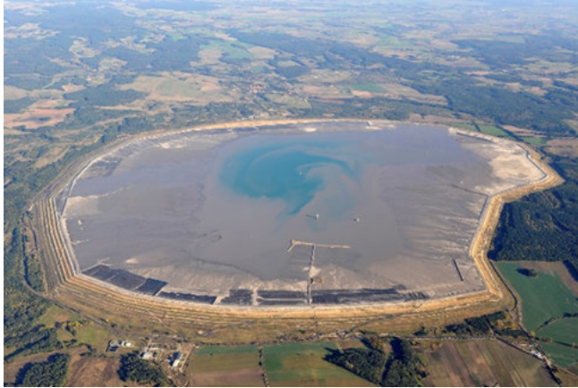
Fig. 1. The Żelazny Most Tailings Storage Facility
