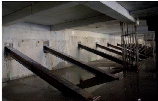
Fig. 1. View of the concrete slurry wall with supports and some construction elements that may obstruct surveying
