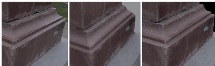
Fig. 8. Plinth. Model from Agisoft PhotoScan, model from VisualSFM and CloudCompare
