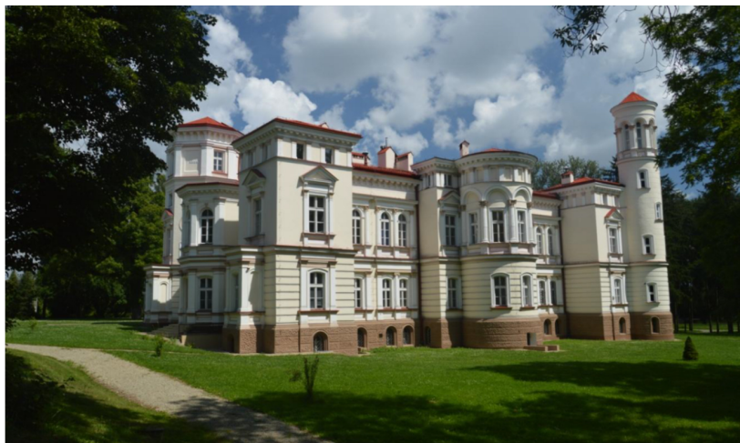
Fig. 2. View of the southern facade of the Lubomirski Palace in Przemyśl
