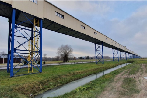
Fig. 2. View of the central segment (2600 m) from the north-east side
