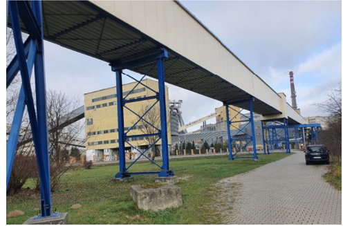
Fig. 3. View of the segment near the industrial plant (300 m) from the south side
