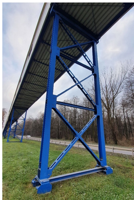
Fig. 6. Swingarm support structure
