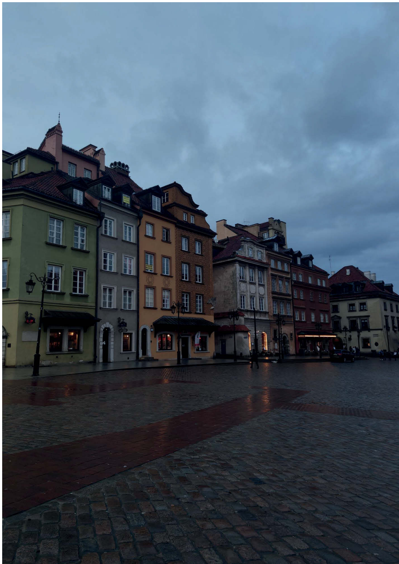
Ill. 1. Rebuilt old tenement houses in the Old Town of Warsaw. Photo by O. Ivashko.
