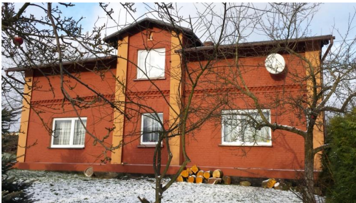
Fig. 15. Southern wall of the building # 3 (Source: own study)
