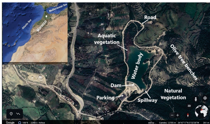
Fig. 1. Satellite map of Boudaroua reservoir and their entourage; source: own elaboration based on Google maps
