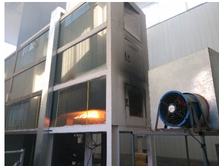
Figure 6: The southern side of the experimental house.
