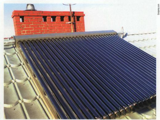
An evacuated-tube collector - this module contains 30 evacuated tubes
