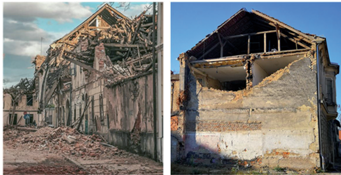
Fig. 1. The Petrinja center immediately after the earthquake in December 2020 (left) and after the removal of debris in October 2021 (right)
