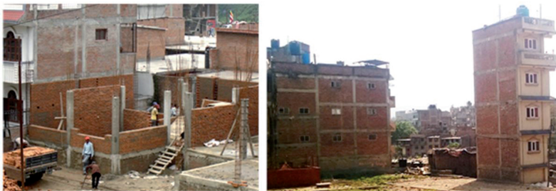
Fig. 6. Structures of buildings in seismic areas made of reinforced concrete frames with brick infill walls (Bhaktapur, Nepal – 2016)
