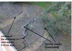
Cracks of the cone of the road bridge abutment in Wronki
