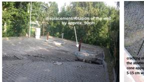
Damages visible at the sewage pumping station of the Municipal Enterprise in Wronki
