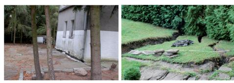
Visible inclination of the building by about 25 cm towards the river in the closed wastewater treatment station of the Correctional Facility in Wronki
