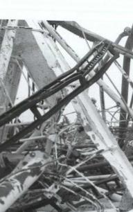
646.38 meters tall, the antenna came online in 1974. Conservation work that was begun in 1991 disturbed the statics of the antenna core, which collapsed on 8 August 1991. The job of broadcasting Polish Radio 1 was taken over by two antennas in Solec Kujawski near Bydgoszcz, only 330 and 289 meters tall
