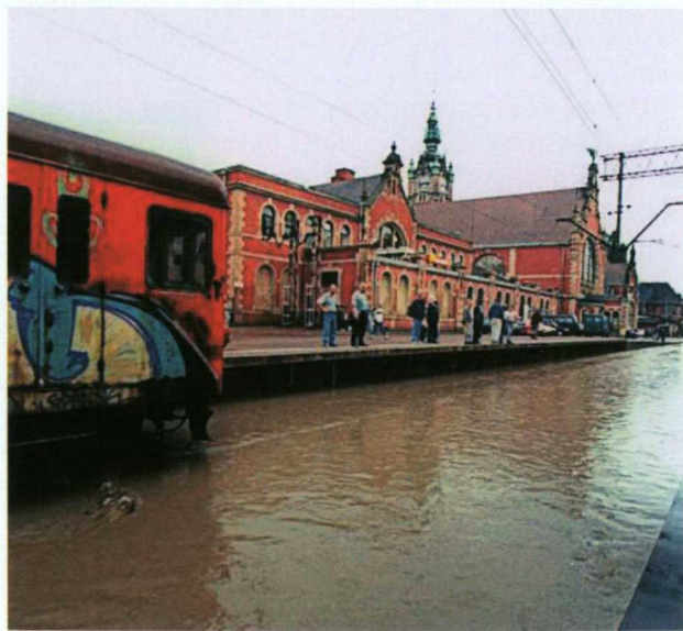
The inundated main railway station in Gdańsk
