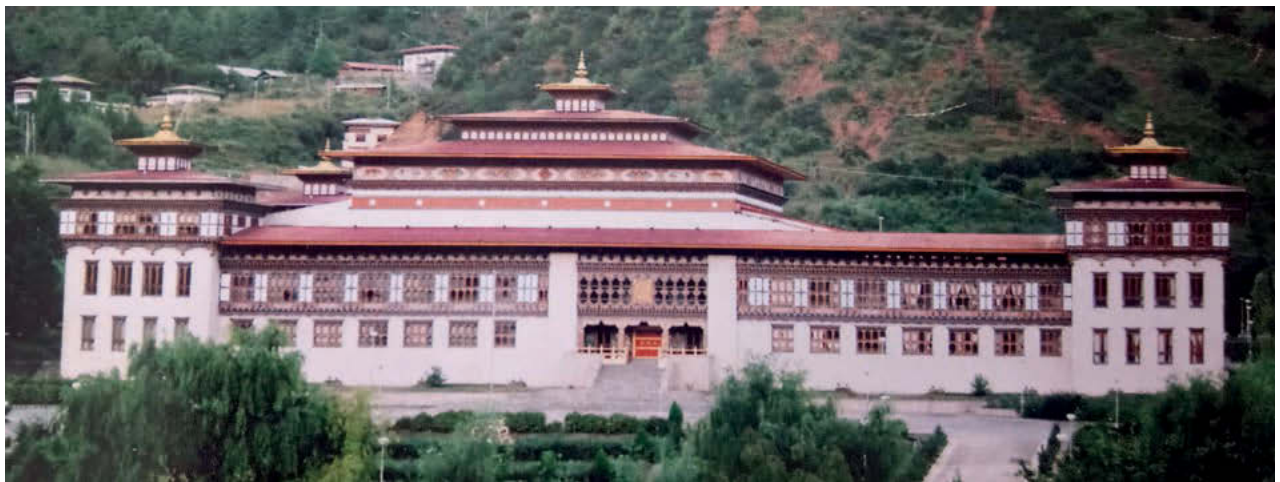
Ill. 8. Bhutan, Dzong, religious and administrative centre. The pent hip roofs emphasise the important function of the building, setting it apart from its surroundings to make it visible from a distance. Photo by K. Sobczyńska.
