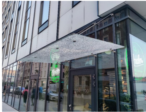
Fig. 1. Glass canopy over building entrance
