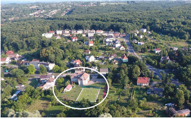
III 4. Primary School no. 2 in Police, marked with an ellipse.
