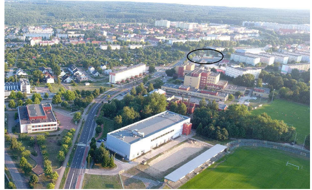
III 5. Primary School no. 3 in Police, marked with an ellipse.
