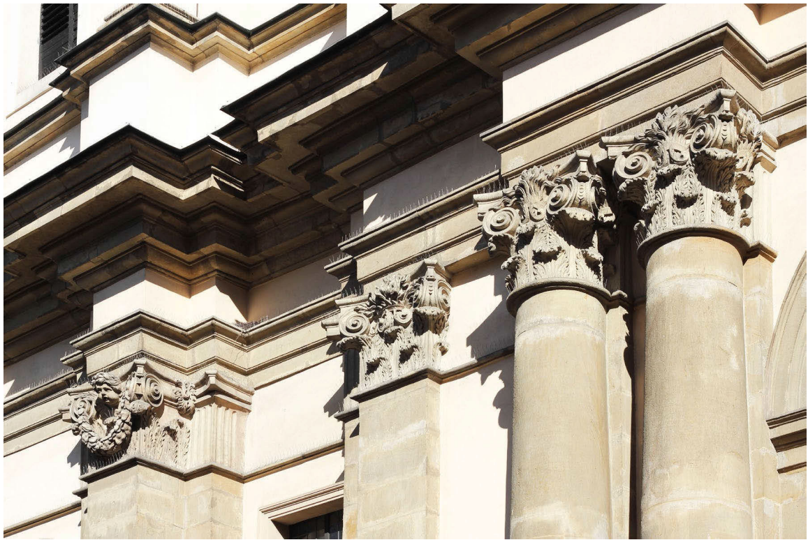
III.1. An example of biomorphism in architectural detail — column capitals and pilasters with ornament depicting acanthus leaves. The University Collegiate Church of St. Anne in Kraków, Photo by J.Białkiewicz, 2024
