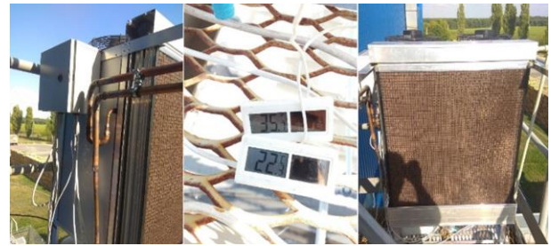
Fig. 8. Liquid subcooler with adiabatic panel.
