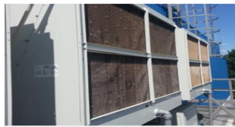
Fig. 6. Air cooled condensers with adiabatic panels.
