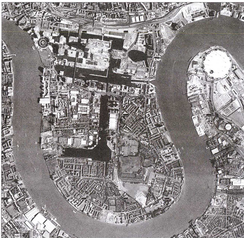
Fot. 8. Canary Wharf
