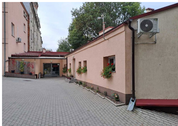
Ill. 8. Implementation in the form of the addition of greenery (climbing plants) on the facades. Original photo.
