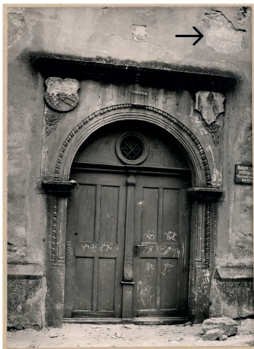
Ill. 7. Złoty Stok, former Corpus Christi church, western portal with visible relic of sgraffito.
