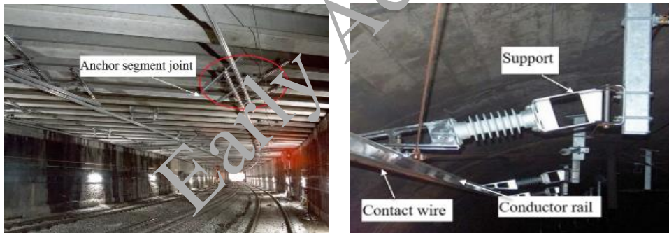
Fig. 1. The anchor section of OCR in the tunnel (left) and its local structure (right)
