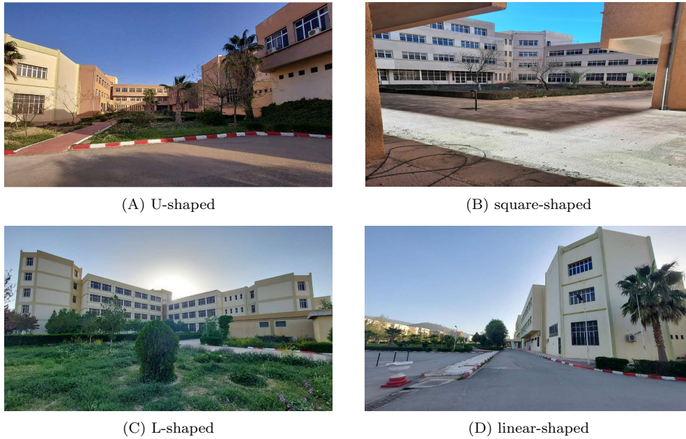
FIG. 2. Photographs of each measurement stations.
