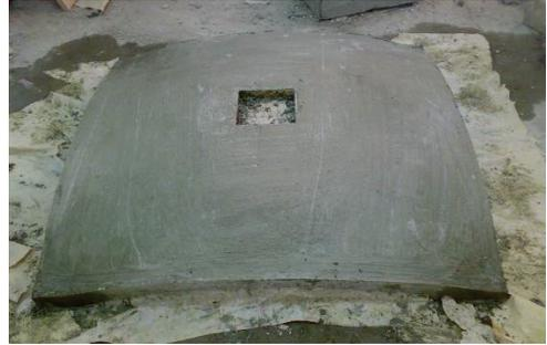
Fig. 2. Shell with central opening.
