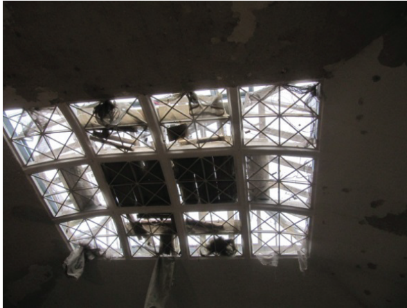
Fig. 4. Reinforced concrete grid of the skylight as seen from the inside of the Seaport Hall
