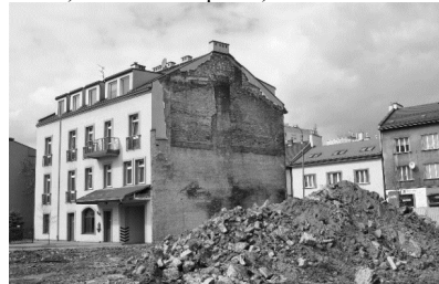
Fig. 6. The segregation of materials from the demolition of the building, Source: own photo, 03 - 04.2014
