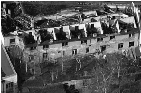
Fig. 3. The top view of the complex of the dry cleaning service "Rainbow" before the demolition, after the fire, around 2012, Source: googlemaps, 06.03.2014]
