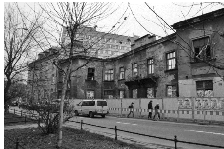
Fig. 4. The view from the Czarnowiejska street on the right wing of the laundry service building "Rainbow", Source: own photo, 06.03.2014
