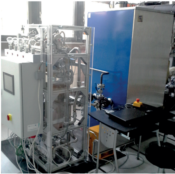
Fig. 6. The prototype of the CHP ORC energy system during the laboratory tests
