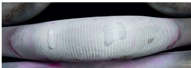
Fig. 17. Cracks after bending repaired by the 141 method
