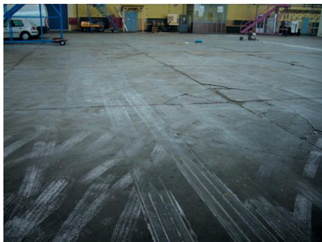
Fig. 2. The hangar slab with visible damages
